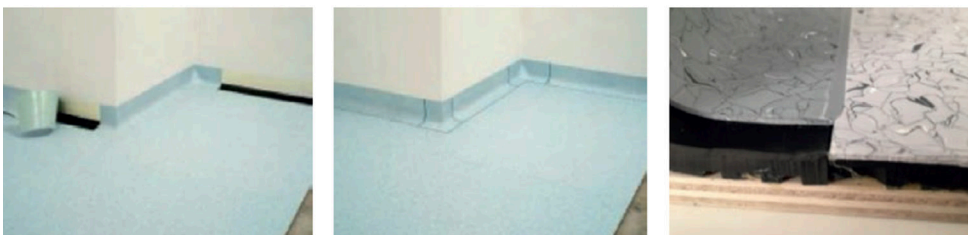
Welded cove former and tile
